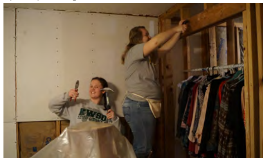
Tori Thorne and Grace Fleming prepare to sheetrock
