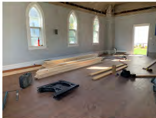
Parish Hall, in progress
