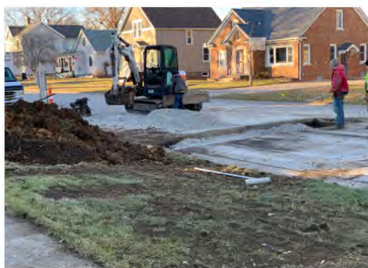
Digging to put in water & sewer for the building
